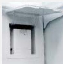
Air purification system.
